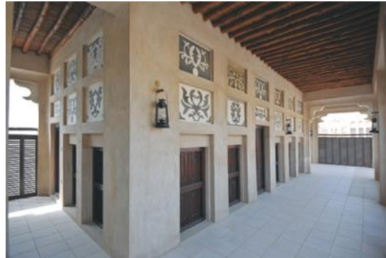
Shape 17 shows ornamented claddings
